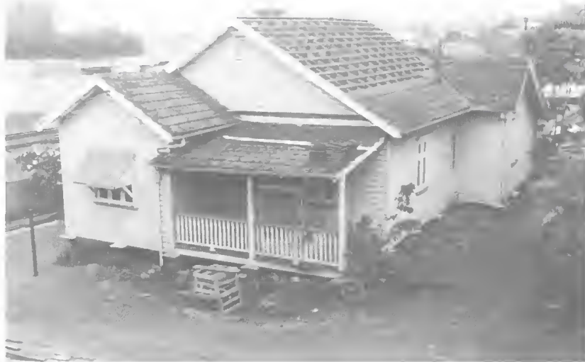
Demolition of the caretaker's cottage near the railway line, 1973. The site was used later as a car park.
